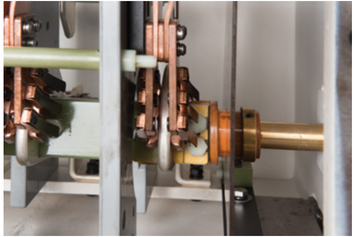
Primary switch contacts and rotor
