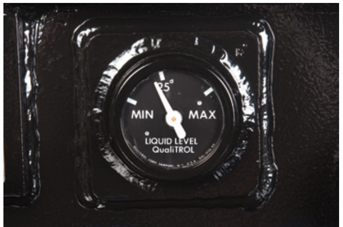
Main tank liquid level gauge
