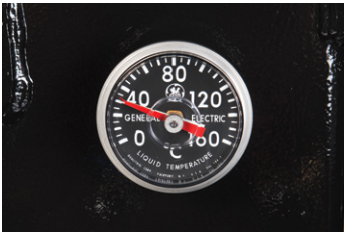
Main tank thermometer
